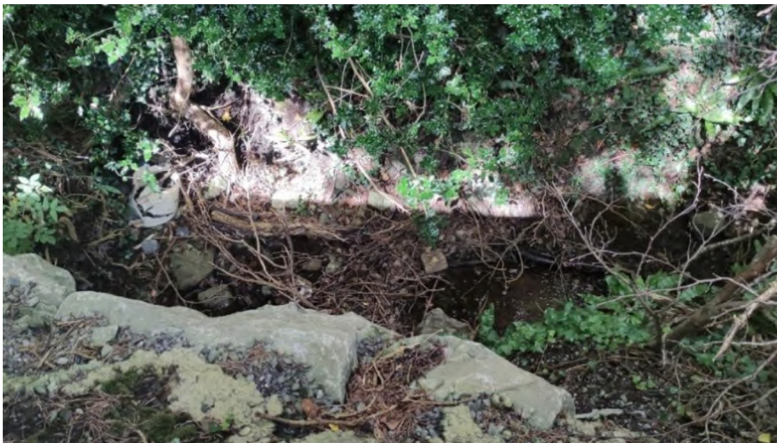
Plate 3-30 Watercourse crossing point number 6
