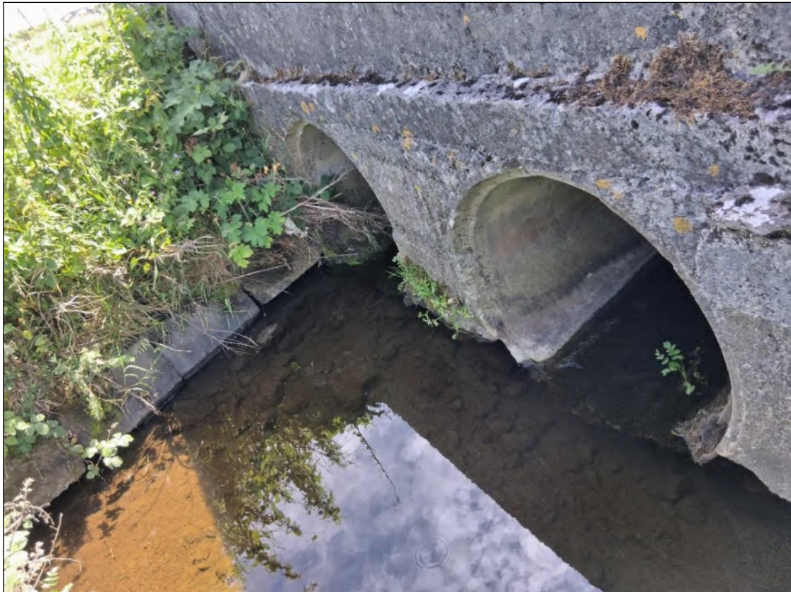
Plate 3-26 Watercourse crossing point 2 from the entrance of the Proposed Project over the Forty Acres Stream
