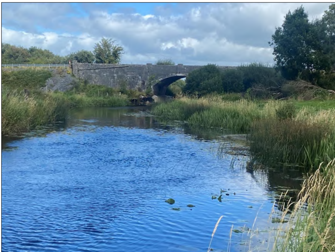
Plate 3-33 Side view of watercourse crossing point 8
