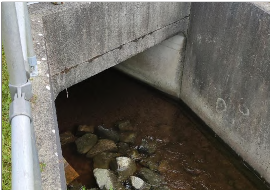
Plate 3-27 Watercourse crossing point 3 beneath the N63, at the Forty Acres Stream
